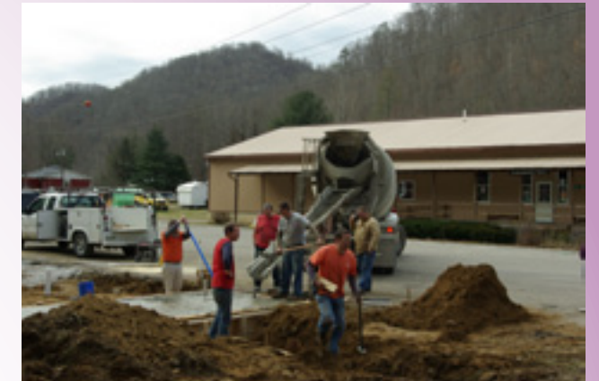
Construction begins on kiosk
